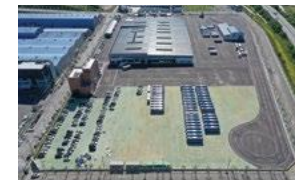
Gimcheon EV Bus Factory
